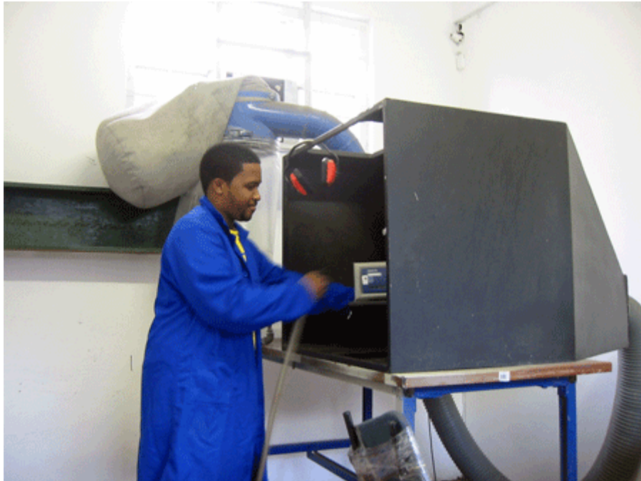
The dust extraction machine at FreeComGroup, Cape Town, South Africa.
